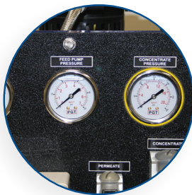
Liquid Filled Panel Mounted Concentrate Pressure Gauge
