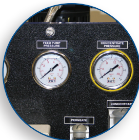
Liquid Filled Panel Mounted Concentrate Pressure Gauge
